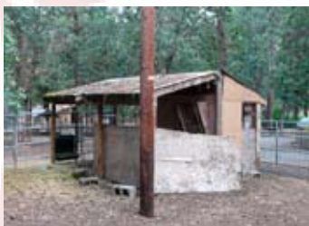
The old pump house
